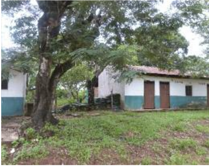
Abandoned police station in El Porvenir
